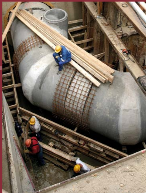
■ PESTERZSÉBET, BYPASS COLLECTOR SEWER, 2010
