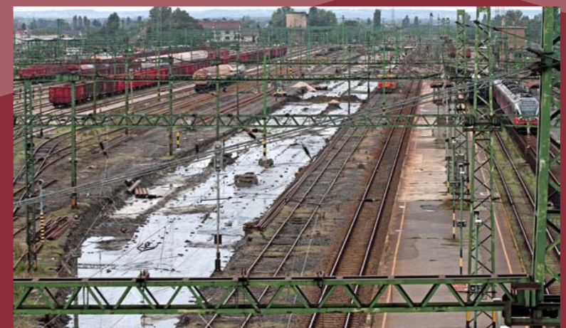
■ M60 MOTORWAY, 2010 ■ SZÉKESFEHÉRVÁR RAILWAY HUB, 2014
