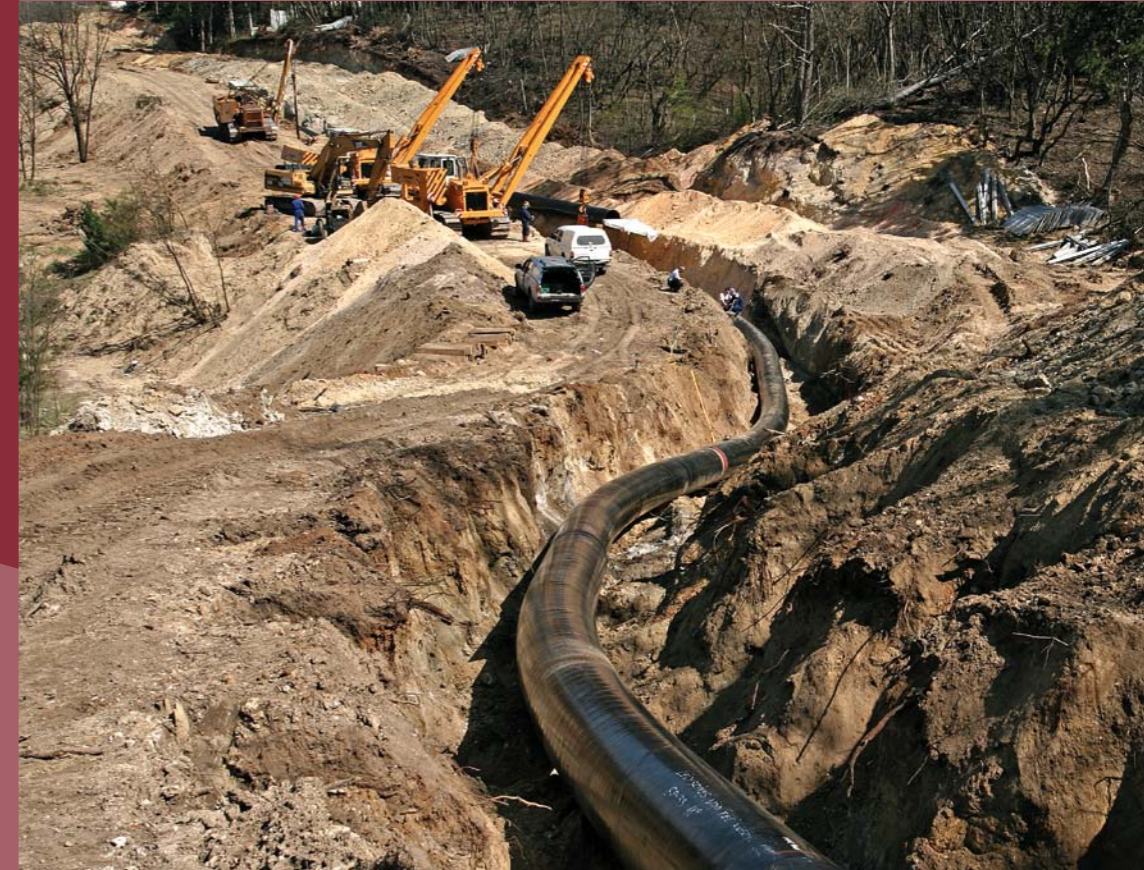
■ PILISCSABA, GAS PIPELINE CONSTRUCTION, 2008
